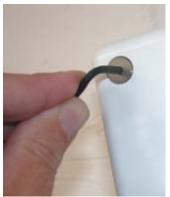
Screw the head screws down with the 3mm allen key provided. Your wiring should be flush and not flattened by tightening down screws.
