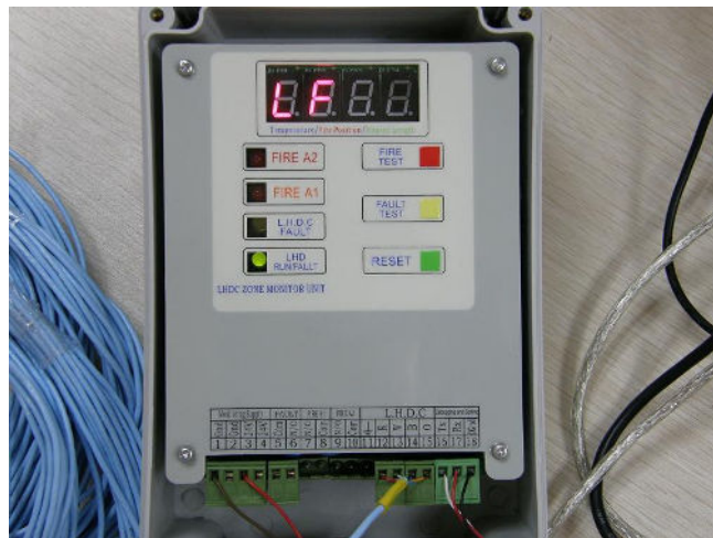
Figure 11.2 – Power on MCU
